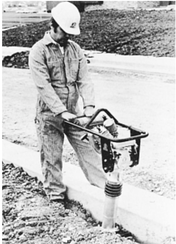
Figure 5-6 Small vibratory rammer. (Courtesy of Wacker Corp.)
