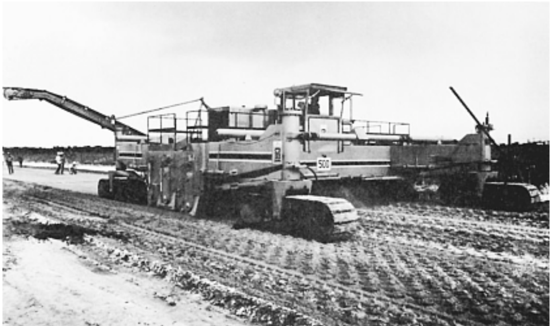
Figure 5-17 Large grade trimmer/reclaimer/paver. (Courtesy of Terex Roadbuilding)
