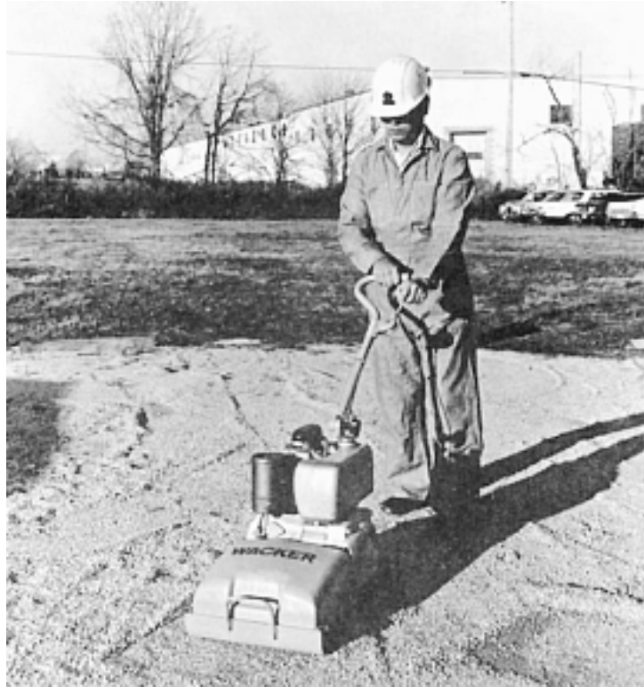
Figure 5-4 Walk-behind vibratory plate compactor. (Courtesy of Wacker Corp.)
